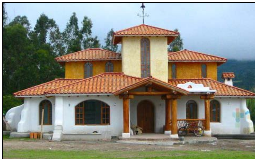
Tapial, or rammed earth custom home under construction
